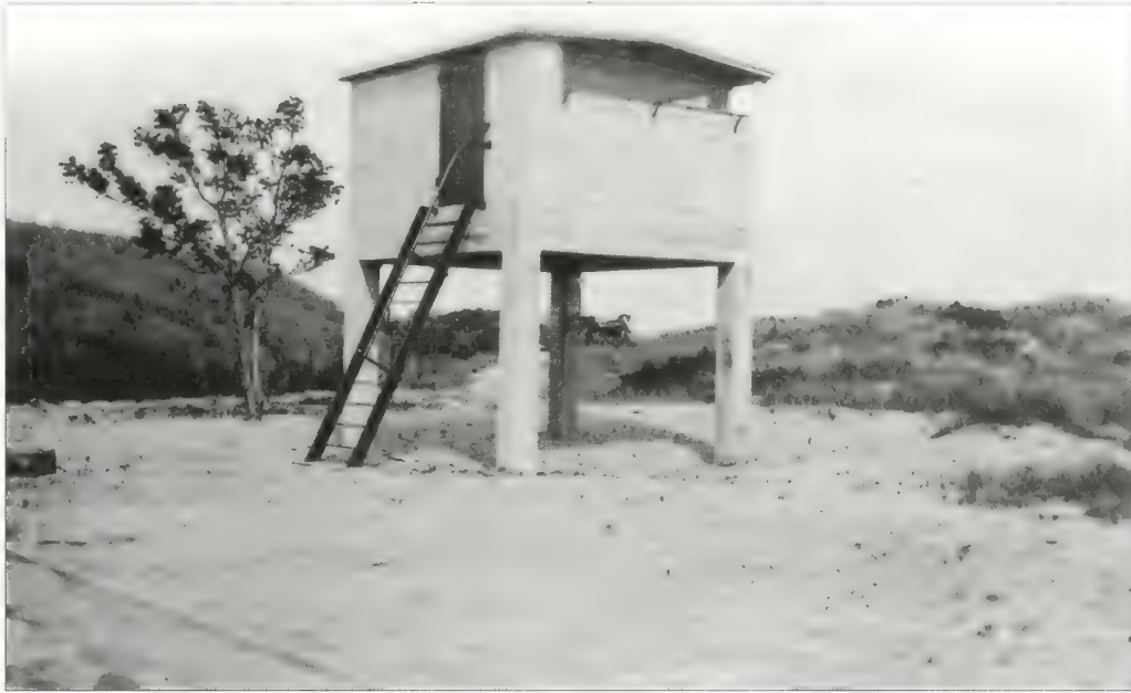
Figure 5.29. Coincidence range finder station, Battery Morris, circa 1920. Note the open character of the adjacent landscape. Woody vegetation should be removed within four feet of the freestanding structure (GATE 7893).
